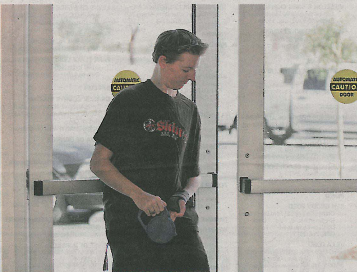
Keith Minnicks, who does not have the use of his left arm, demonstrates the door equipped with "panic bars" that can be opened with a push at AbilityFirst apartments in Irvine. > oc post
